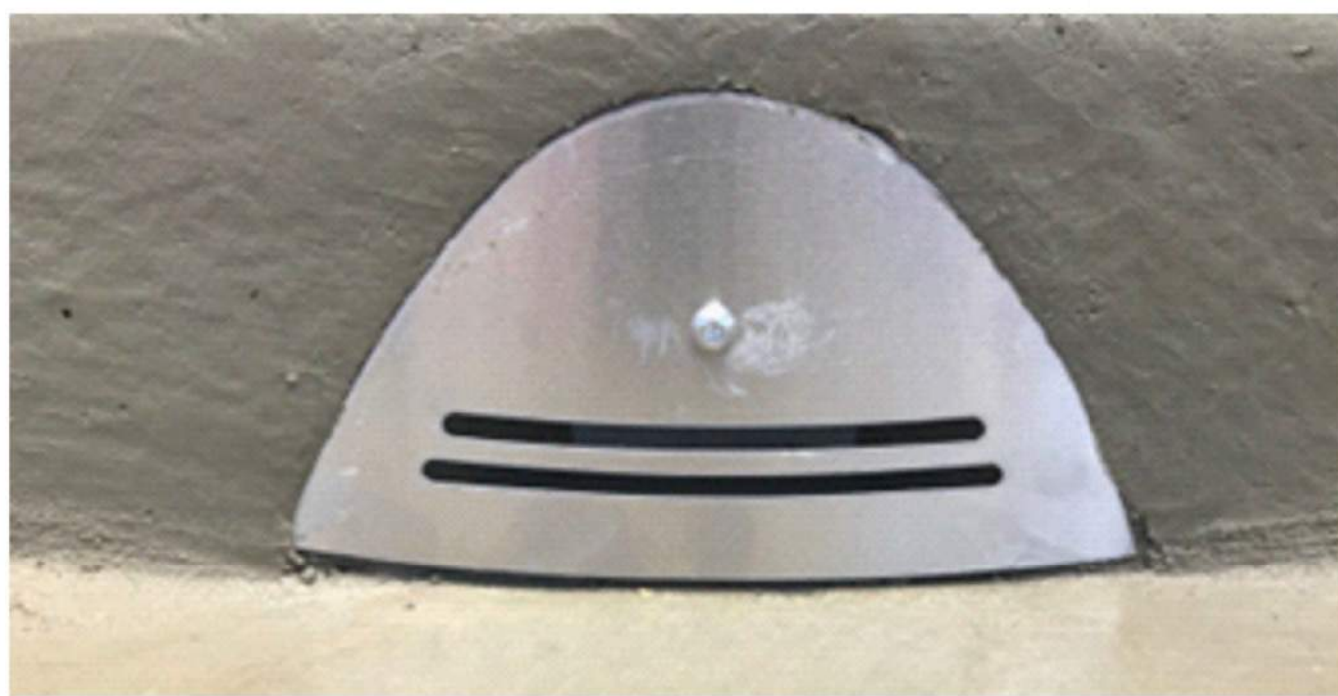
FIGURE 1 TREENET R750 KERB INLET (OR EQUIVALENT)
