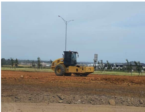
Photograph 7: Vibrating Pad foot compacting clay
