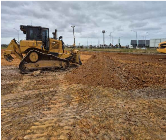
Photograph 5: Dozer spreading clay
