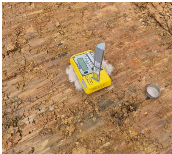
Photo 10: PNDG Field density/moisture test
