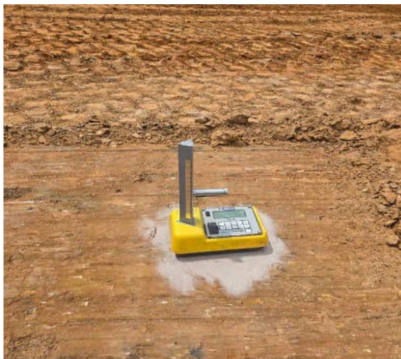
Photo 9: PNDG Field density/moisture test
