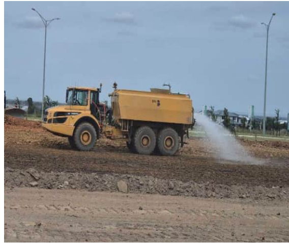
Photograph 6: Water cart conditioning clay
