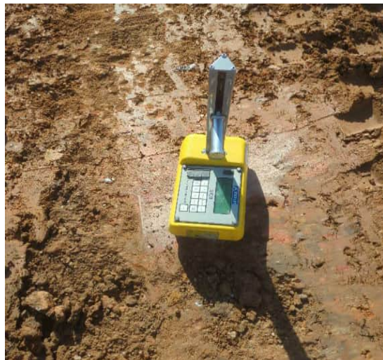
Photo 10: Field density/moisture test
