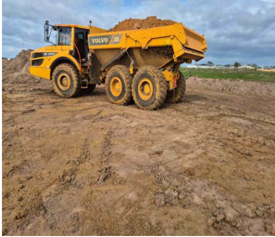
Photo 3: Subgrade assessment with Dump truck
