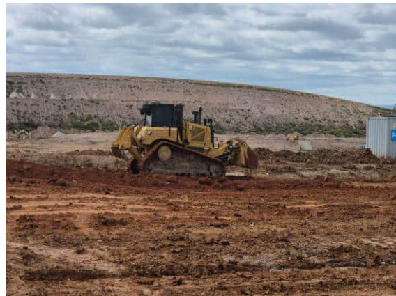
Photograph 8: D6 Dozer spreading fill
