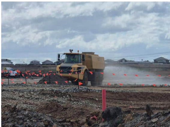
Photograph 7: Water cart conditioning clay
