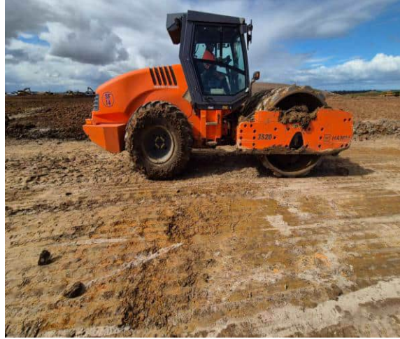
Photo 4: Subgrade assessment with pad foot
