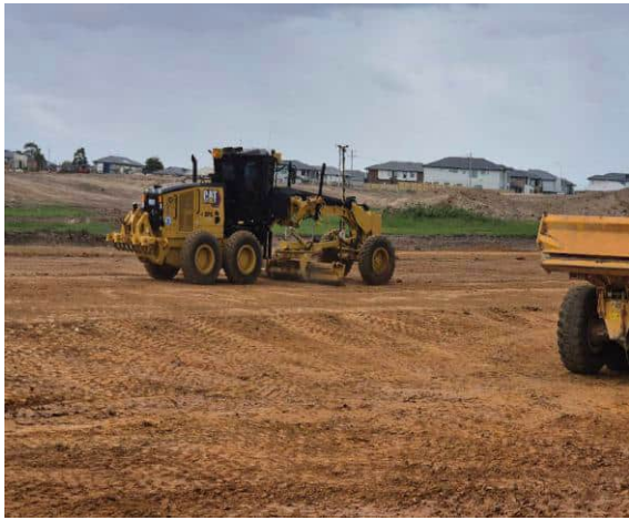
Photograph 5: Grader trimming surface
