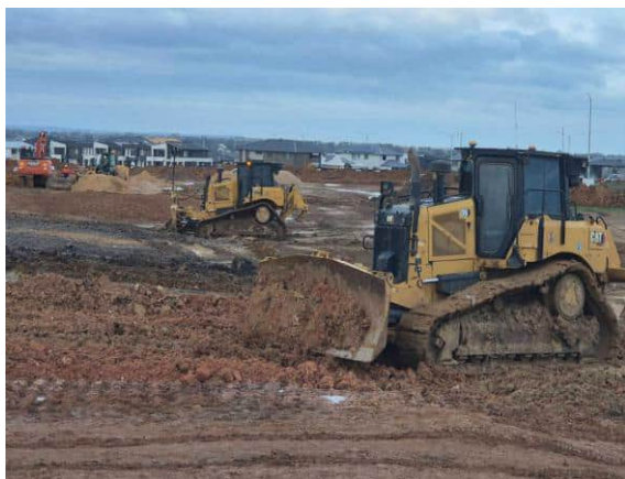
Photograph 5: Dozer spreading clay fill material.
