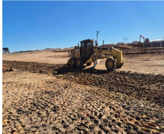
Photograph 8: Grader ripping.
