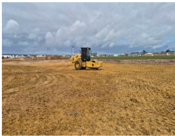
Photograph 6: Vibrating Pad foot compacting
