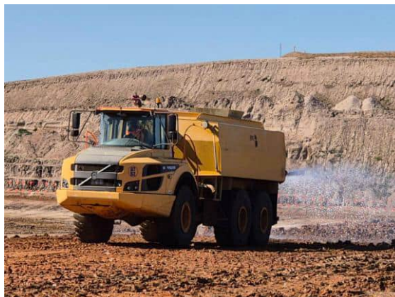
Photograph 8: Water cart moisture conditioning
