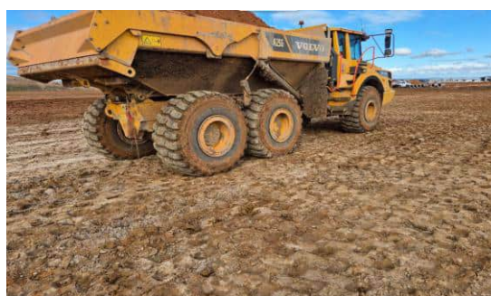
Photograph 4: Subgrade assessment with a loaded dump truck
