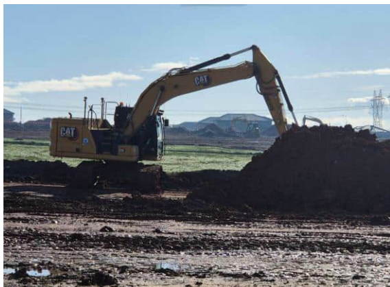
Photograph 7: Excavator spreading clay.
