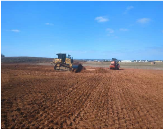
Photograph 5: Pad foot Roller compacting.
