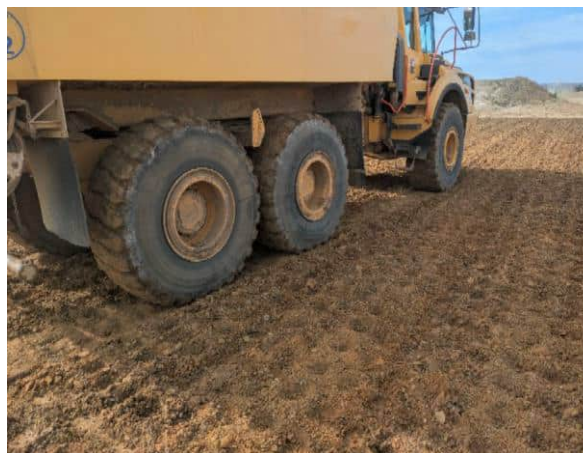
Photograph 4: Subgrade assessment with a loaded water cart
