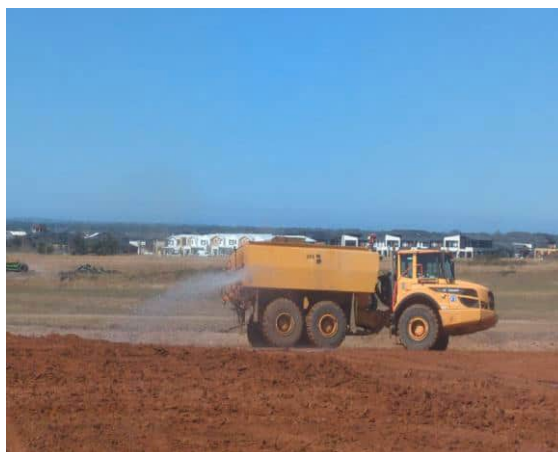
Photograph 6: Water cart moisture conditioning
