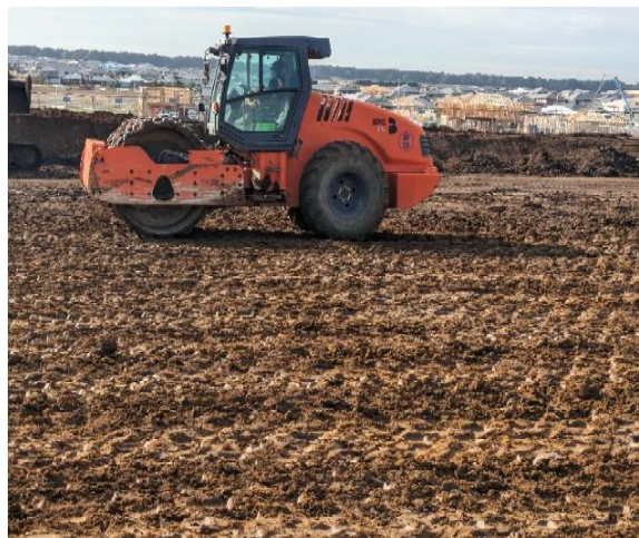
Photograph 4: Subgrade assessment with 15 Tonne Pad foot Roller
