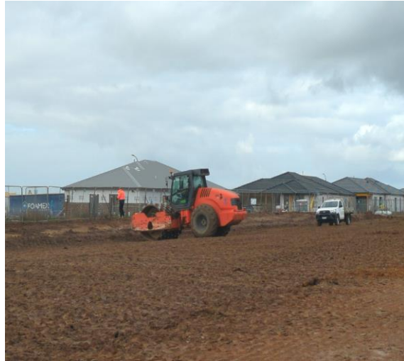
Photograph 8: Pad foot compacting fill material
