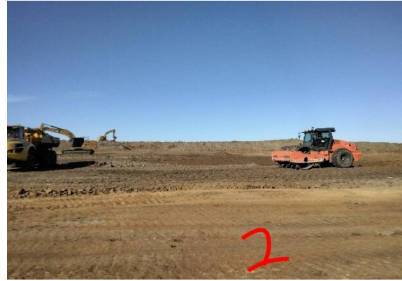
Photograph 2.7.2: Compaction with Padfoot
