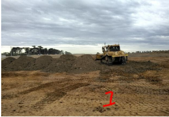
Photograph 2.7.1: Material Spreading and placement
