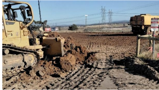
Photograph 2.7.2: Material placement
