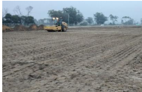
Photograph 2.2: Material compaction, March 2021
